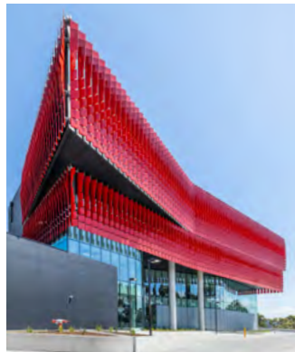
M2 Melbourne 75 Sharps Road, Tullamarine VIC 3043
