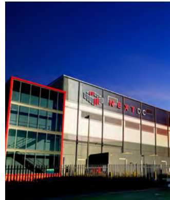
P1 Perth 4 Millrose Drive, Malaga WA 6090
