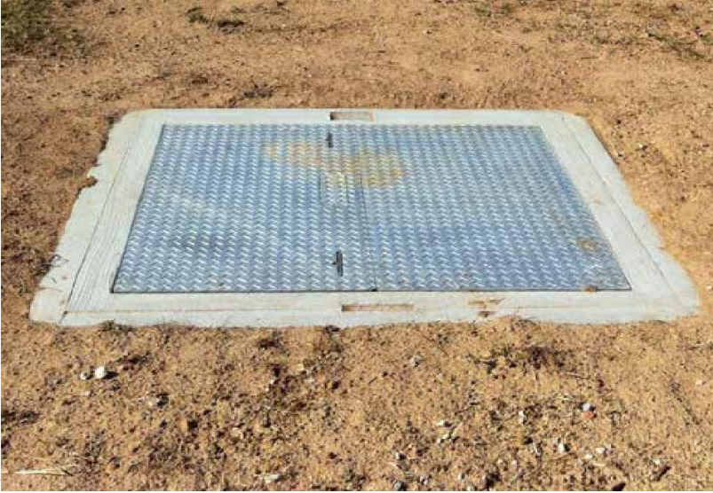
Concrete/Steel Draw Pit at Facilities other than B1.
